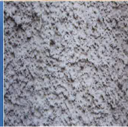
Walling and Slab Edges
