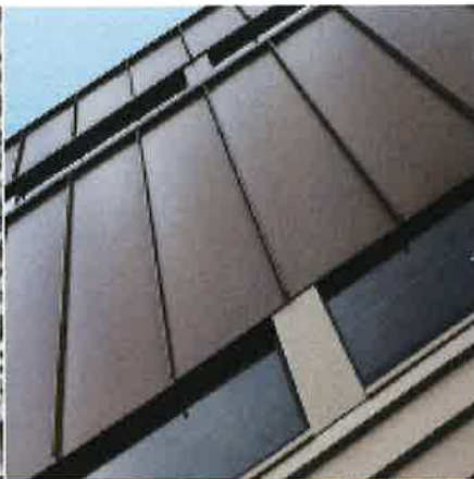
Walling and Eaves Colorbond Jasper Standing Seam
